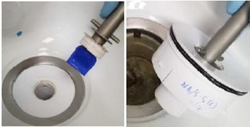
Figure 3 - Sumpless Cartridge Style with Silicon Check Valve (2 Months Operation)
